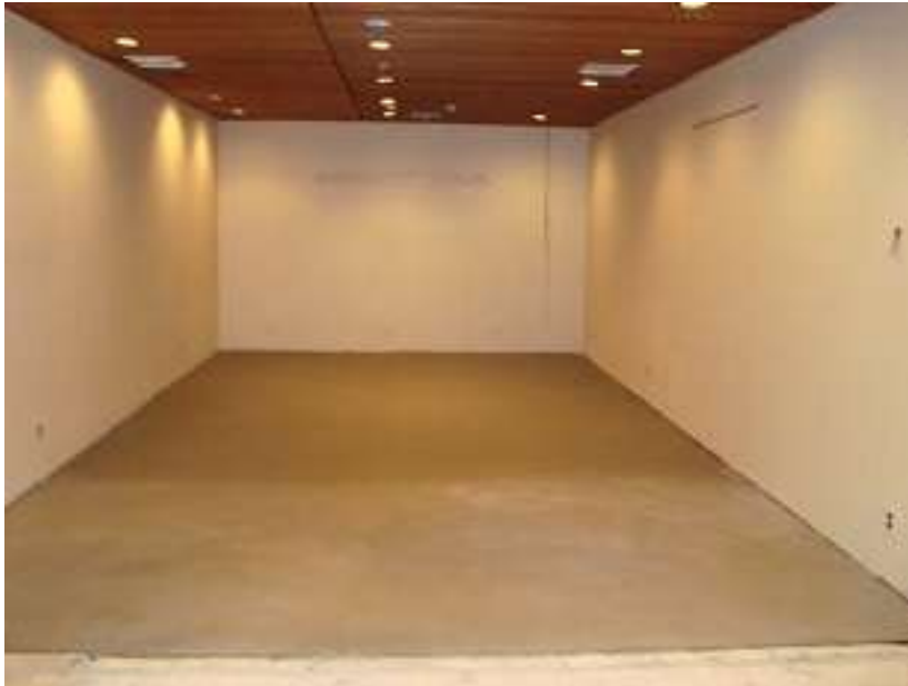
new Paoli Room raised floor
