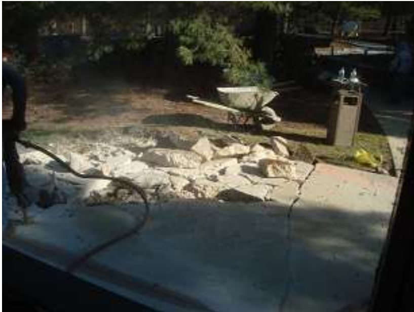
removal of concrete by Main Level entrance
