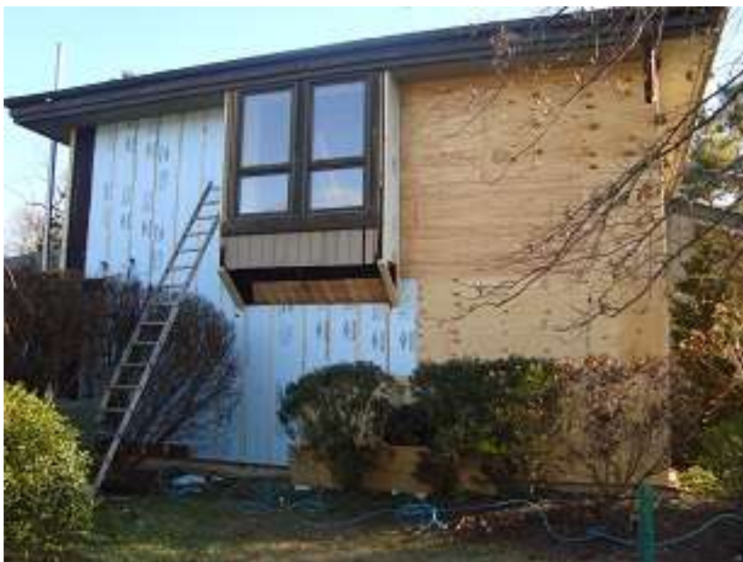
adding blue rigid insulation to 2 story exterior walls
