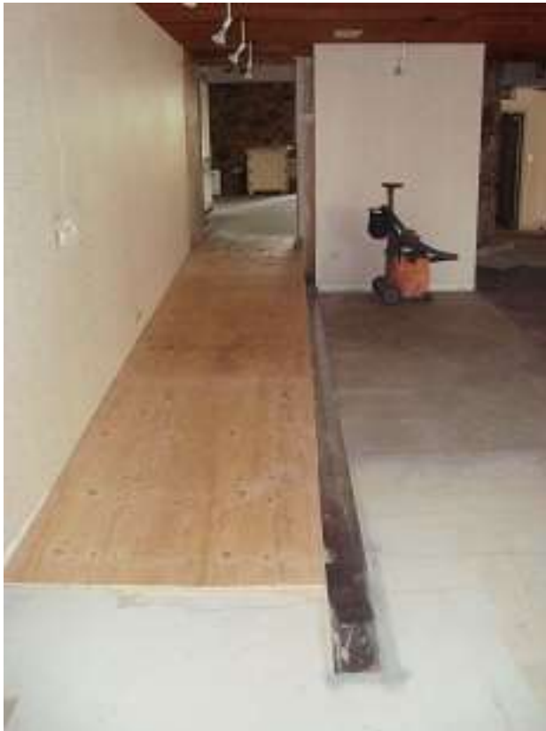
looking up new ramp from Paoli Room
